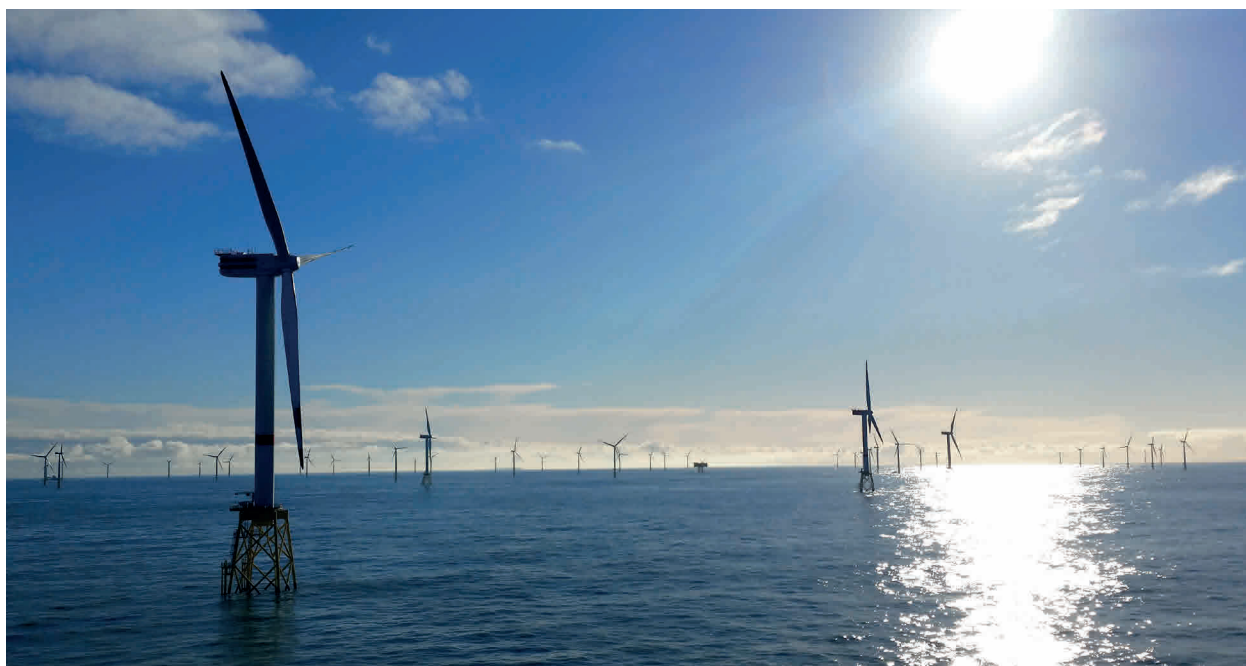
Sun and wind – a good combination. Freudenberg favors both solar and wind power.
