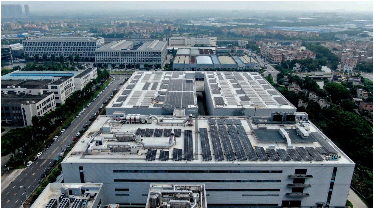
The array consists of roughly 38,000 individual solar panels – making it one of Freudenberg’s largest.
